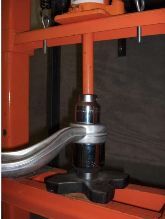
1. Press out the stock bushing using the appropriate bushing press and driver. For reference, the following Sears/Craftsman sockets will work as the driver and receiving cup:
